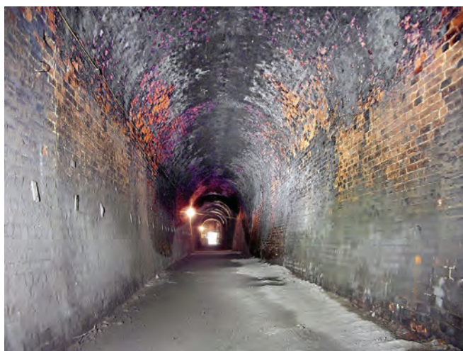
Looking west along the tunnel. Photo Ade Armishaw
